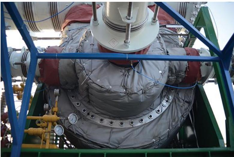
**2. Dual-drive.** Shown here installed on the Akca Tosunlar plant, the radial outflow turbine takes the working fluid through the center of the disk. The vaporized fluid flows outward and exits out the sides. Using only a single turbine disk means fewer rotating components and a smaller footprint for the plant as a whole. *Courtesy: Exergy*
